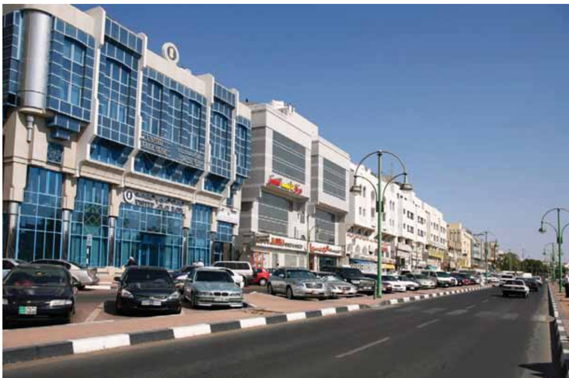
Economic development in Al Ain can be accommodated by the versatile G+4 typology that mixes residential, retail and office space into a seamless whole
